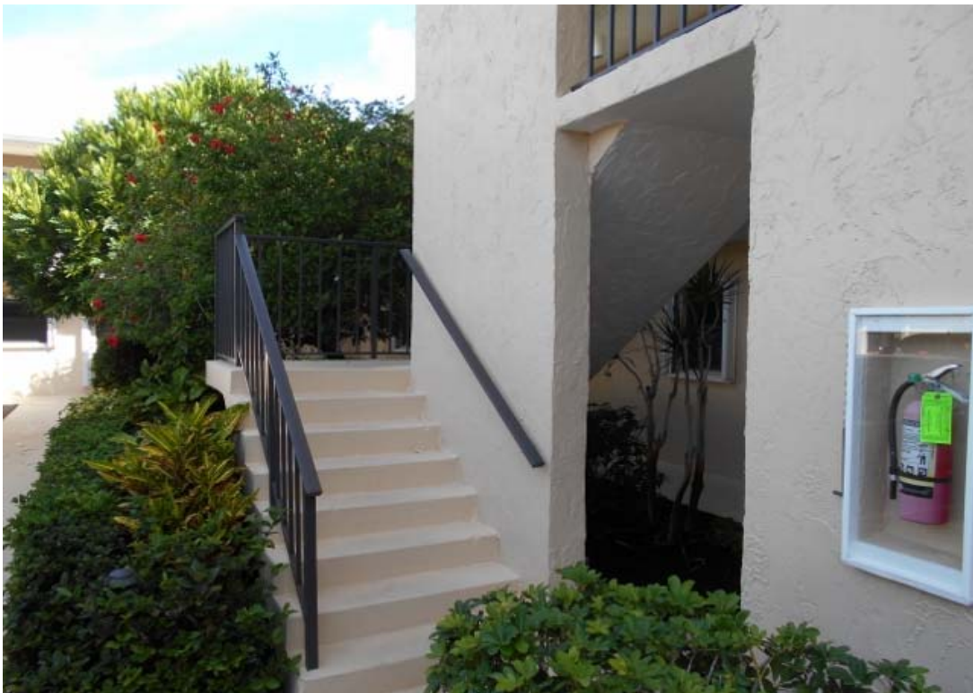
TYPICAL VIEW OF SUBJECT APARTMENT STAIRWELL
