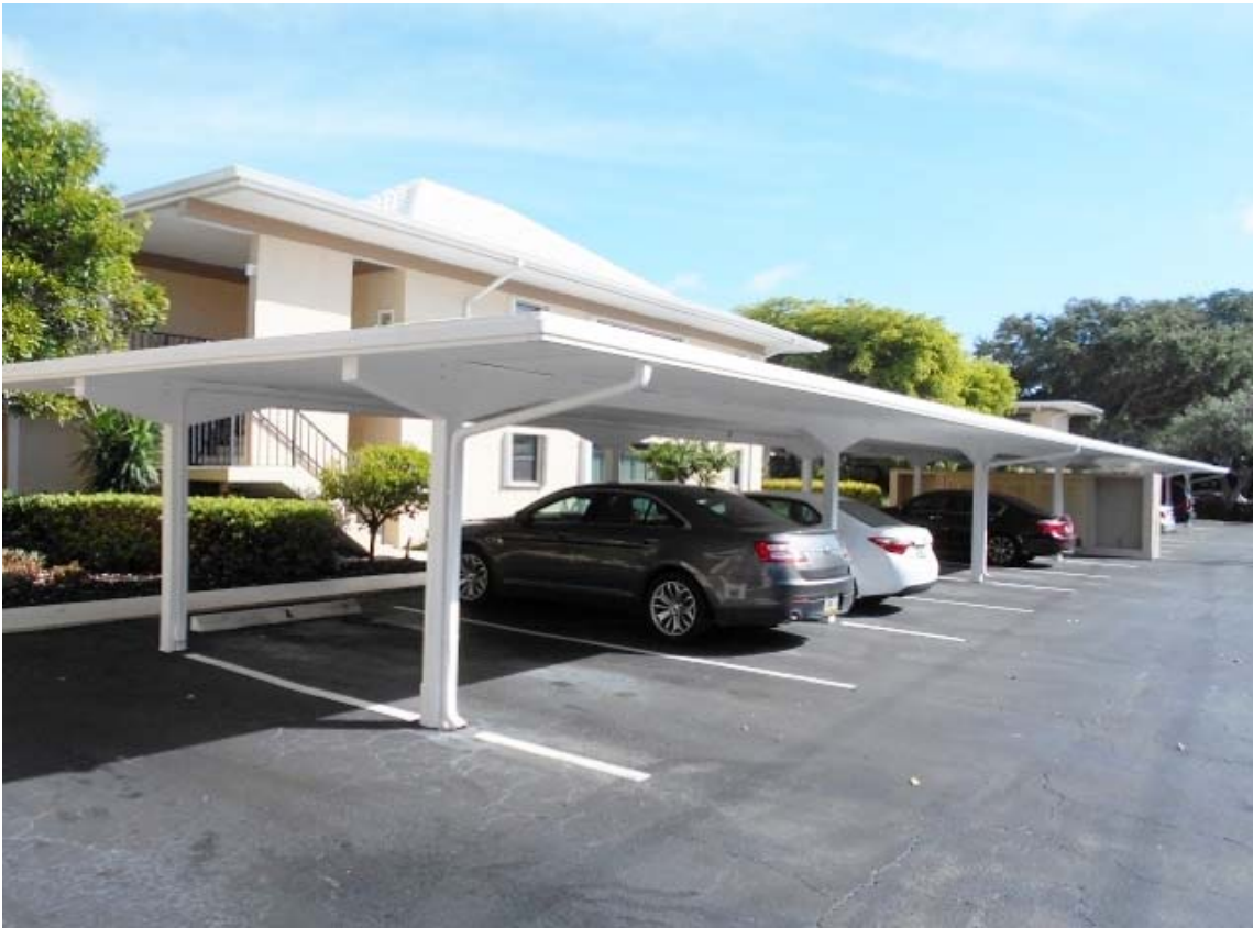
VIEW OF GALVANIZED STEEL CARPORT
