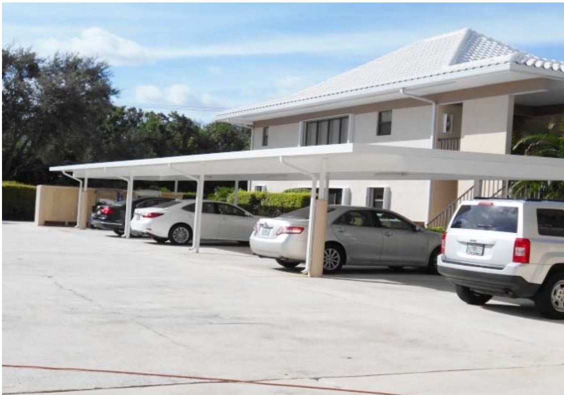
VIEW OF ALUMINUM CARPORT
