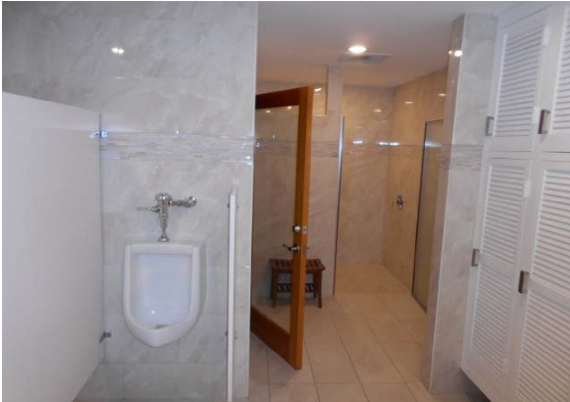
TYPICAL VIEW OF SUBJECT RESTROOM/LOCKERROOM
