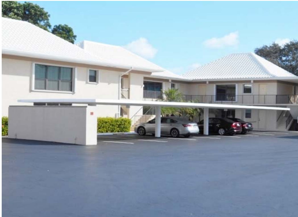
TYPICAL VIEW OF SUBJECT APARTMENT BUILDING AND CONCRETE CARPORT
